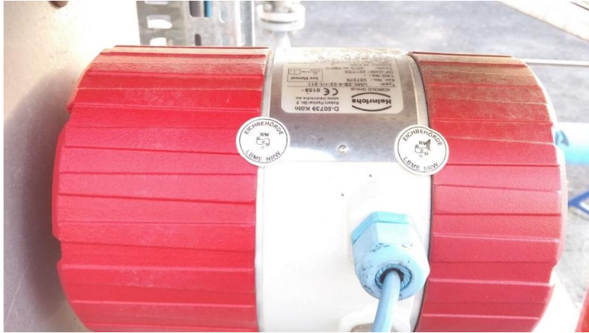
Image 1: Seals on the transmitter covering the lid and rating plate
